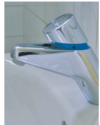
Our toilets are equipped with automatic taps and economic flush knobs. Photo by Claudia Wagner
