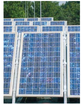
In 1999, teachers and pupils installed our first photovoltaic (PV) system. Today, we wish to expand our PV system in co-operation with local craftspeople. Together, the new and old solar panels could back feed a maximum of 8kW of excess energy to the grid. Photo by Michael Meier-Hahn
